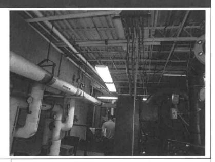
The 30-plus year old chiller serving Building 36 failed in the spring of 2016. MEI was retained to design the installation of a temporary rental chiller, which remains in service at this time. MEI was then retained to design a full HVAC retrofit to the building due to the condition of the air handlers, ductwork, VAV boxes, and associated systems. The building presented unique challenges as it was originally two buildings in which the common space
