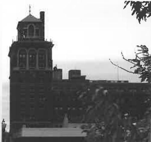
McKinley & Associates' Washington, PA Office
