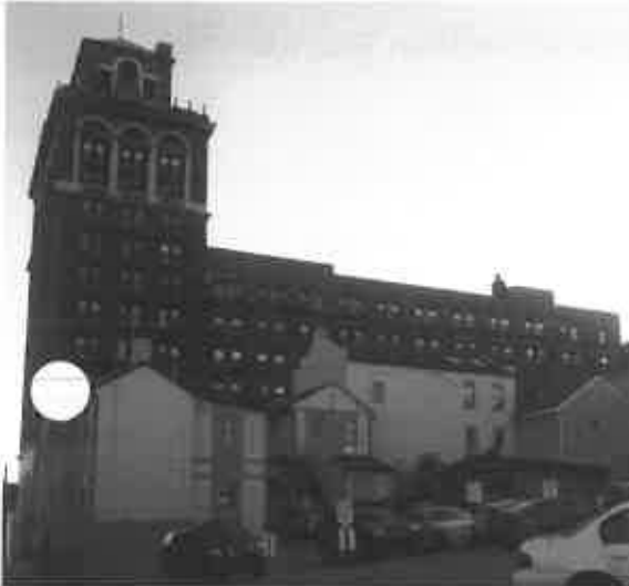
McKinley & Associates' Washington, PA Office
