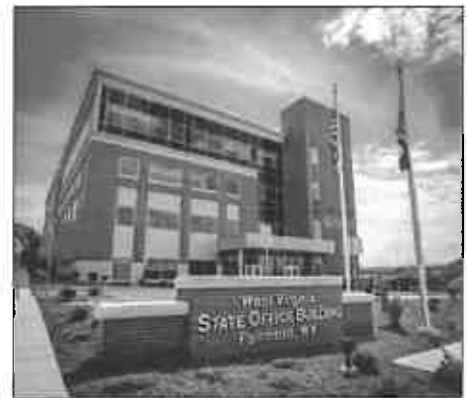
West Virginia State Office Complex Fairmont, West Virginia
