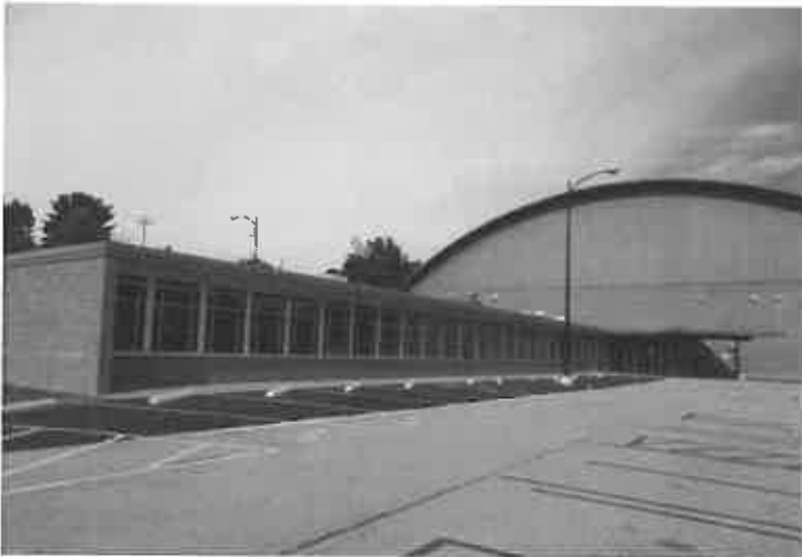
MARION COUNTY BOE OFFICE RENOVATIONS Fairmont, WV
