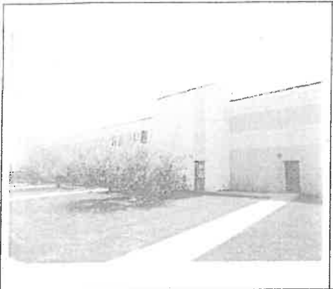
Front View of Structure
