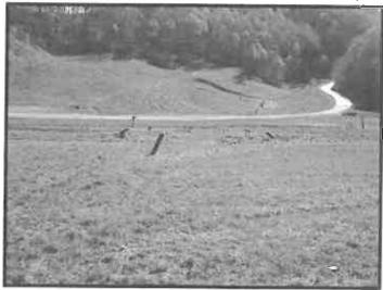
The intent of the proposed closure plan systems was to; minimize surface water infiltration, thereby minimizing generation of leachate, collect and remove any surface and/or subsurface leachate seepage, collect and remove gas generated during waste decomposition, and to minimize the potential for erosion of the closure cap by surface water run on/runoff.
