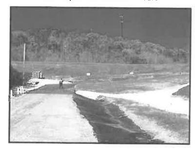
Albans, West Virginia. Construction Quality Assurance/Quality Control monitoring and materials evaluation were also performed by Triad. The repairs consisted of collecting and properly sealing seeping waste and leachate and repairing the access road.
