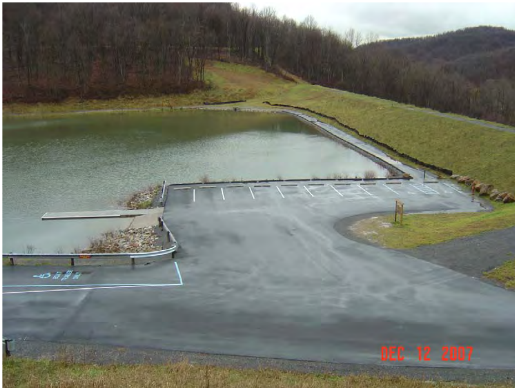
BAILEY DAM MODIFICATION, MONONGALIA CO., WV
