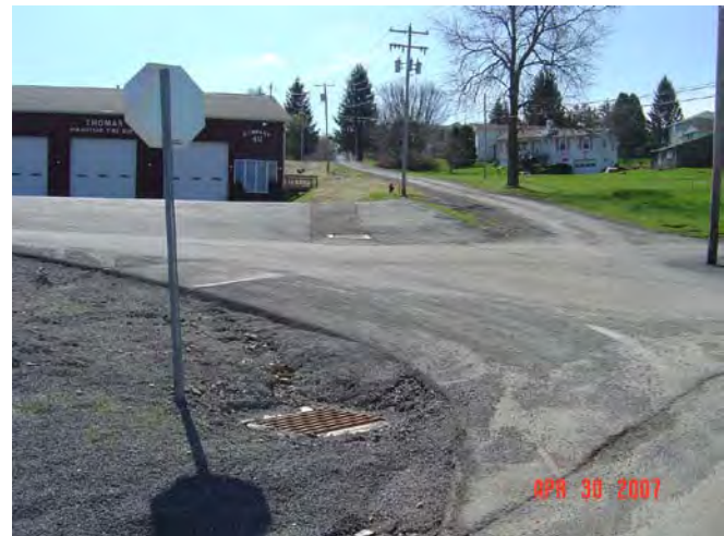
New Storm Drains and Catch Basins
