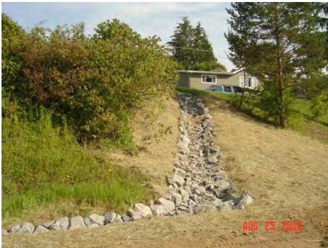
Erosion Repair – Rip Rap Armored Ditch
