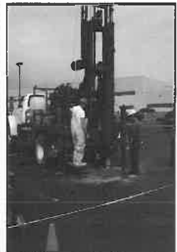
Drilling on Flat Terrain
