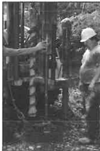
Drilling in Rough Terrain
