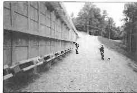
Finished wall with anchors
