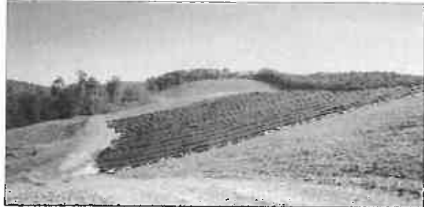
Cell 1-B slope covered with geosynthetic cap prior to placing the final soil cover layer.
