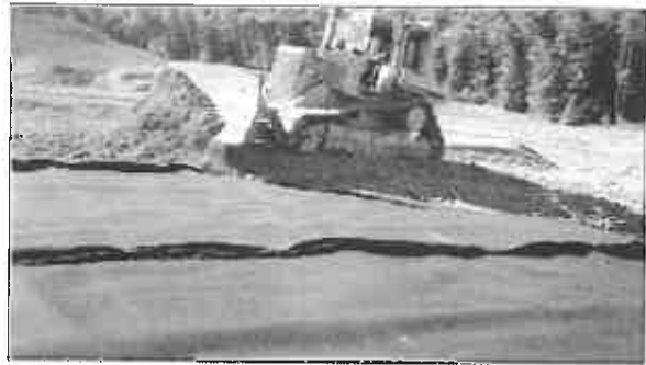
A bulldozer was used to place the 2-foot thick final soil cover layer working from the bottom of the slope to the top.
