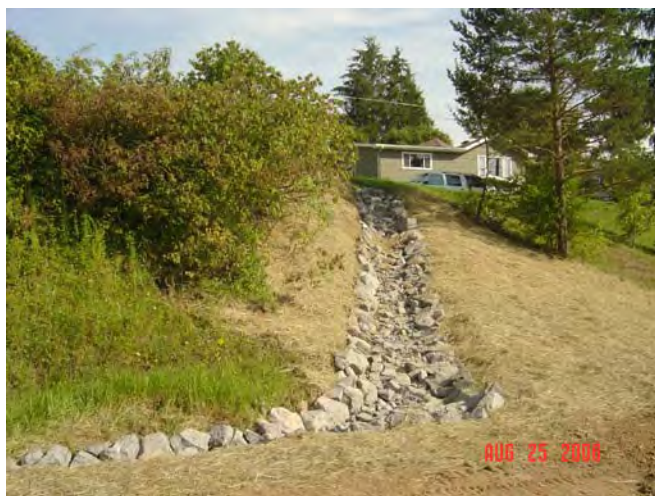
Erosion Repair – Rip Rap Armored Ditch
