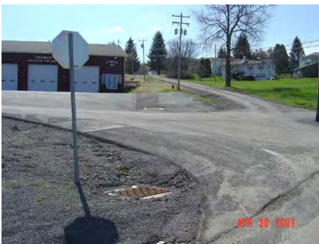
New Storm Drains and Catch Basins
