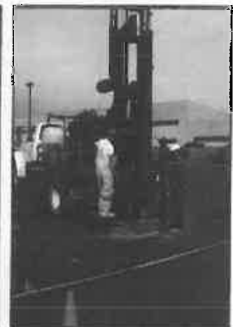
Drilling on Flat Terrain
