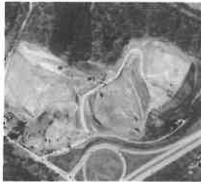
Gateway Development Site: I-79 Exit 155
