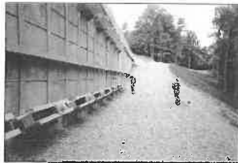
Finished wall with anchors
