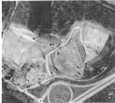
Gateway Development Site: I-79 Exit 155
