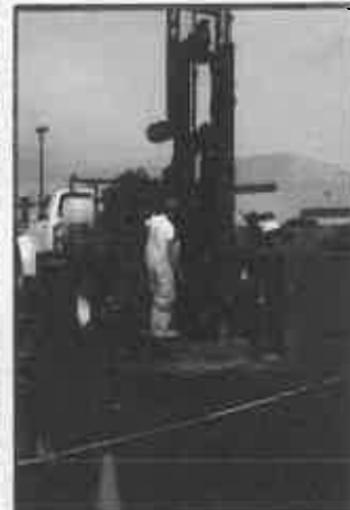
Drilling on Flat Terrain
