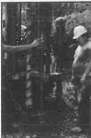
Drilling in Rough Terrain
