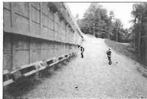
Finished wall with anchors
