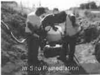
Underground Storage Tank Removal
