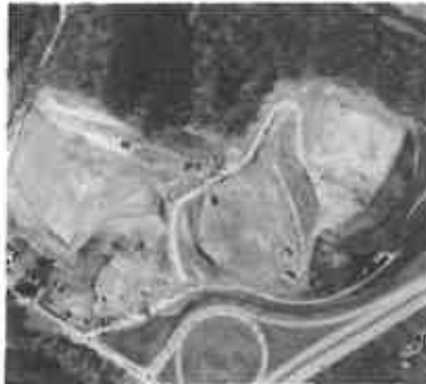
Gateway Development Site: I-79 Exit 155
