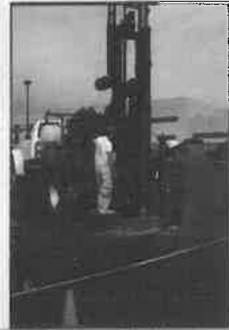
Drilling on Flat Terrain
