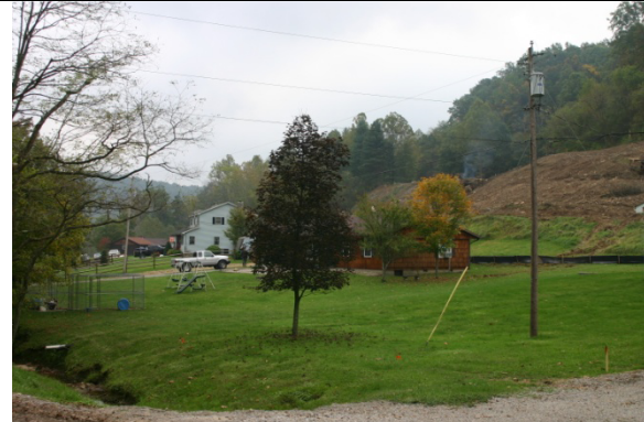
SAULS RUN STRIP AND LANDSLIDE AML related slip threatening residences along Sauls Run
