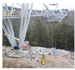
as-built surveys for all underground utilities on site and field surveyed the lines prior to backfill. Additionally TERRADON is developing as-built plans off the survey information to eventually be turned over to the Summit.
