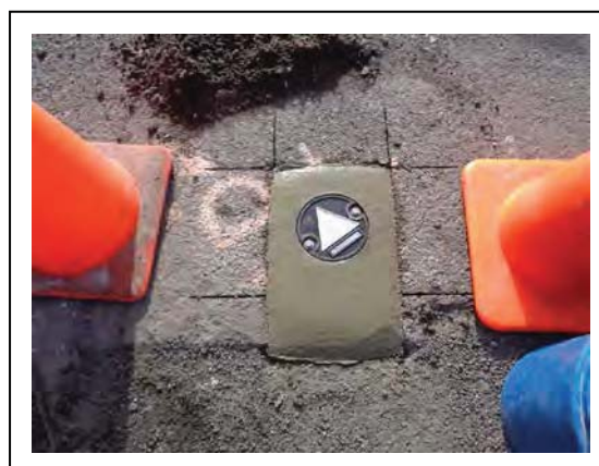
Representative well installation
