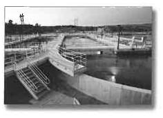
a lagoon to a mechanical treatment system. Tetra Tech provided planning, design and construction administration services for the new plant, which was completed at the end of 2008. The new regional wastewater treatment plant has an initial capacity of 2.50 MGD, expandable to 5.0 MGD. This facility serves the Town of Clifton and outlying communities.
