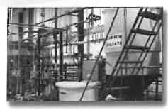
recycling facility in the Village of Dundee with a design flow of 90,000 GPD. The system discharge needed to meet the industrial pretreatment requirements for the village.
