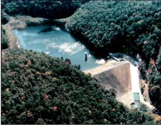
The spillway design flood exceeded the existing spillway capacity. To eliminate this inadequacy, O'Brien & Gere designed a new, ogee-shaped overflow section, side-channel spillway, spillway chute and stilling basin. The computer programs HEC 1 and HEC 2 were used to size the overflow and spillway chute sections. The stilling basin geometry and sizing were selected using criteria established by the U.S. Bureau of Reclamation.
