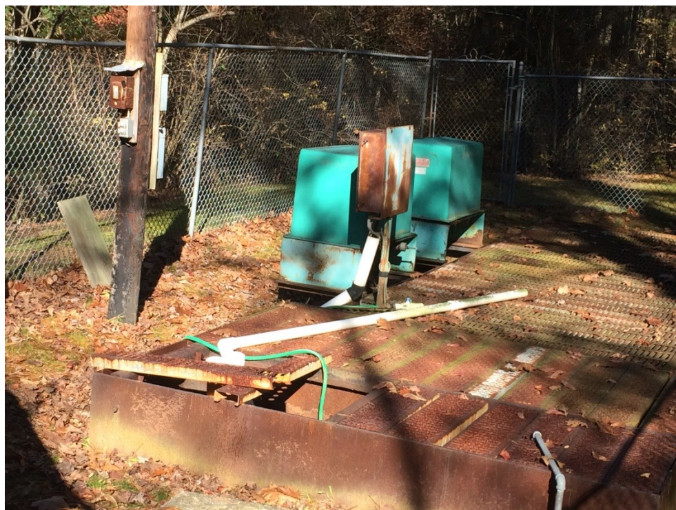
Moncove Lake State Park Extended Air Wastewater Treatment Plant – Sized and Permitted for 7,500 gallons per day (GPD)
