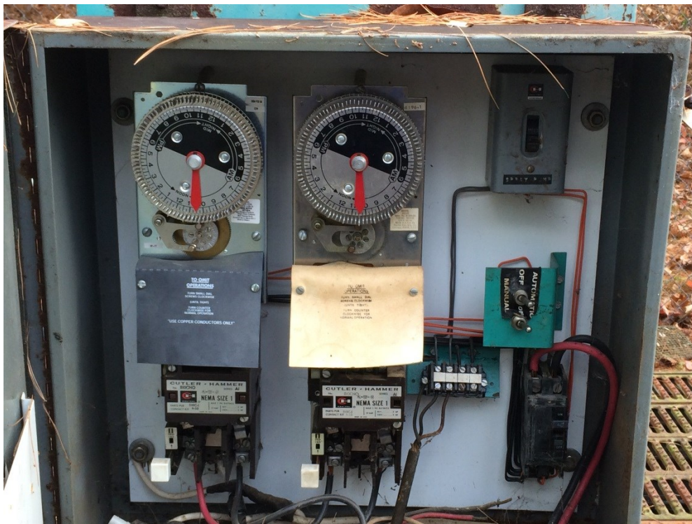
Moncove Lake Controls and Timers – These need replaced and the electrical service upgraded.
