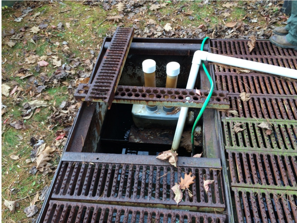
Moncove Lake Tablet Chlorination Feed and Chamber – This should be replaced due to age and condition.
