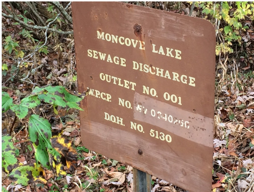
Moncove Lake NPDES No. 0040260 – Shows evidence of washout near the outfall pipe. Consider installing a headwall.
