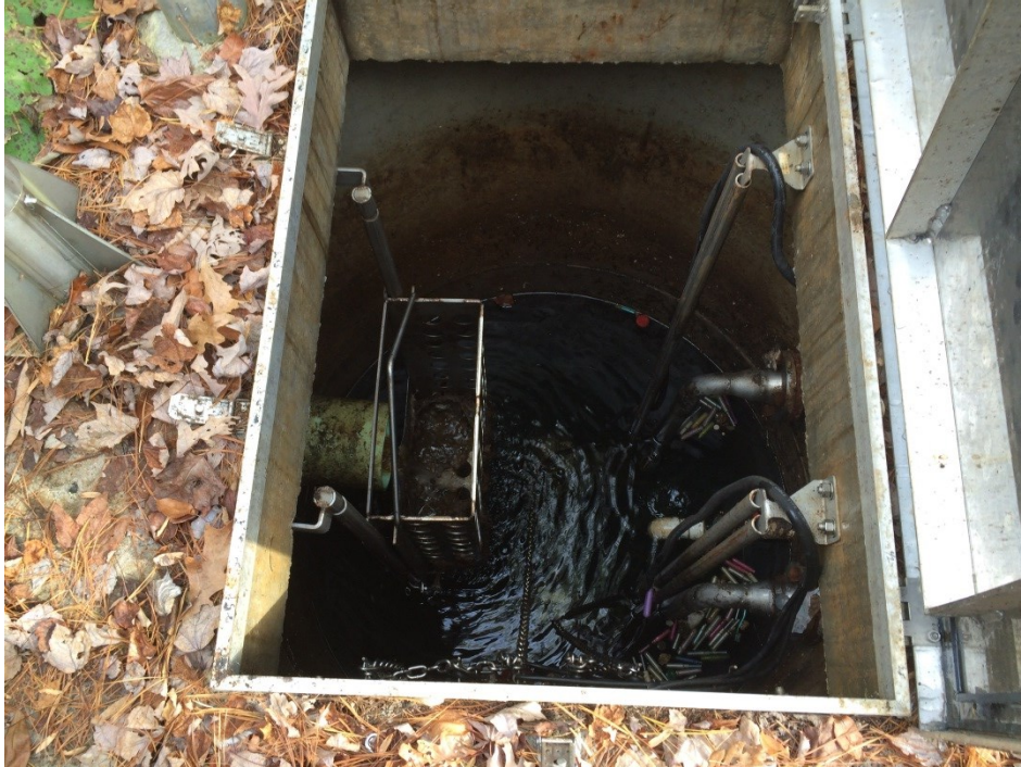
Moncove Lake Pump Submersible Pump Station – Flygt Submersible pumps need retrofitted with grinder pump impellers.
