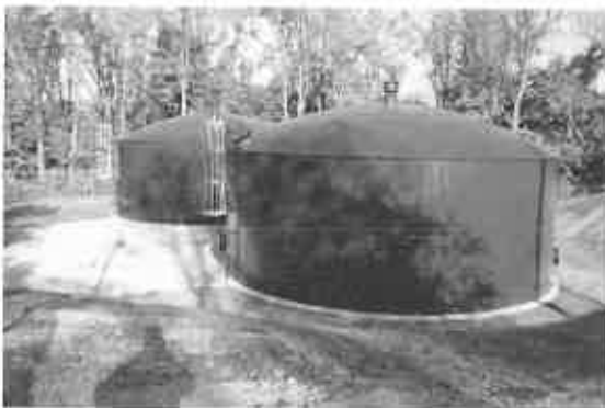
Two new water storage tanks.
