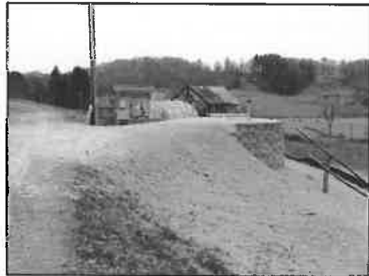
50 GPM Booster Station
