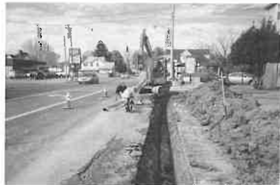
Replacement of water line along US Route 60.
