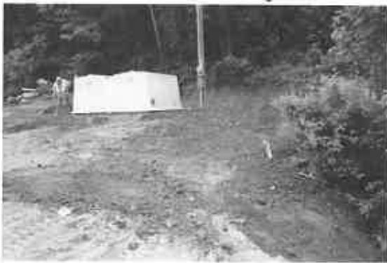
New booster station during construction.
