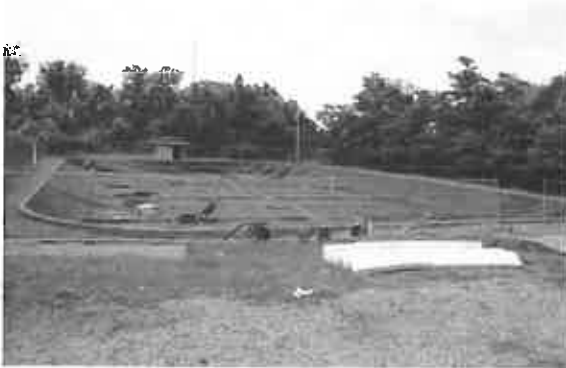
Reservoir Floating Cover Replacement
