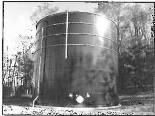
402,000-Gallon Water Storage Tank
