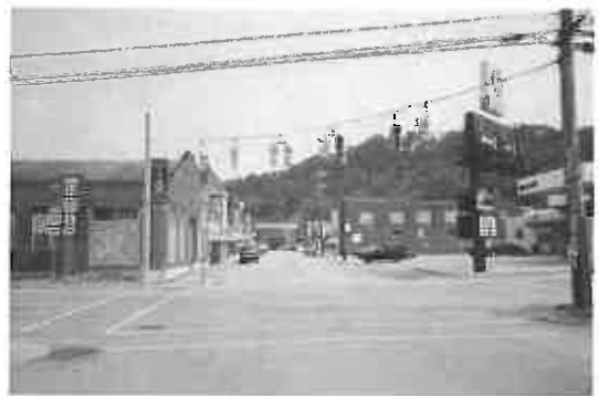
Main Street Where 8" Water Line Was Installed
