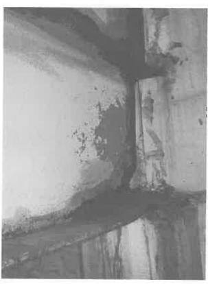
A steel pipe column was added below the bearing end of this beam due to the severe deterioration at the end of the beam.
