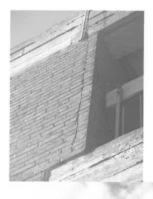
Project included structural repairs to masonry wall. An expansion joint was placed in the roof but never in the wall, resulting in a crack in the wall below the joint in the roof.
