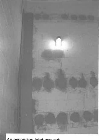
An expansion joint was cut completely through the exterior wall, an angle was installed in the corners of the stair tower and reinforcing steel and grout were installed to reinforce the walls.
