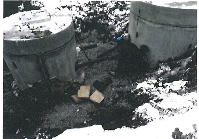
Lift Station Improvements
