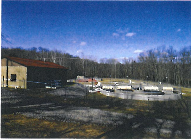
New 0.370 MGD WWTP
