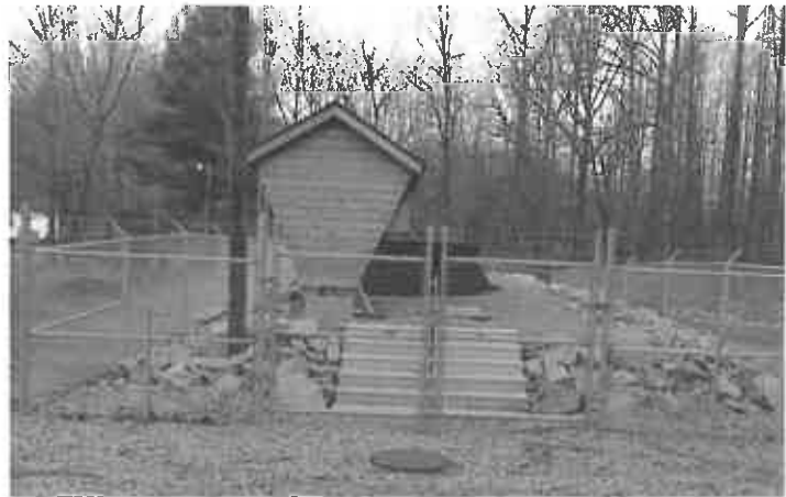
Community of Ury Wastewater Treatment Facility (part of Crab Orchard-MacArthur PSD)
