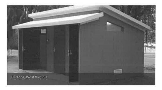
ELR prepared design documents for a prefabricated restroom structure for its site construction and installation within the City of Parsons Mill Race Park along the Allegheny Highland Trail to serve the trail users. The design included ADA compliant sidewalk connections to the restroom, utility connections to the city's sanitary sewer and water lines and underground electrical utility service.
