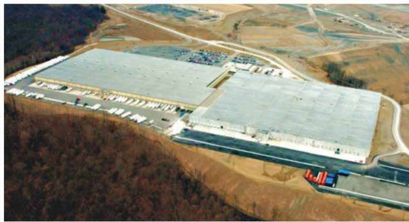
Cabela's Eastern Distribution Center
