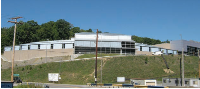
Hilltop Elementary School (LEED Certified)
