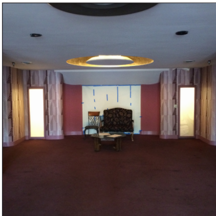
Existing Balcony Lobby
