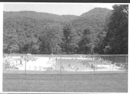
The pool at Bluestone resides within the flood plain of Bluestone Lake and special consideration was required to actually allow the pool basin, if empty at the time, to flood to prevent it from "floating" should the lake level reach the pool. To our knowledge, the approach selected has never been utilized in the area before and was of our own design. The pool had experienced total basin failure and could not be
