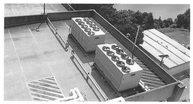
Charleston Civic Center (2015) – Replace entire MEP infrastructure three 1,000 ton chillers and cooling towers, three 8,000 mbh gas condensing boilers, approximately ten VAV AHU's, approximately 10 large single zone VAV AHU's.
