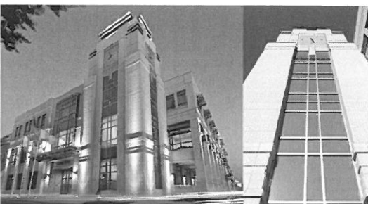
Raleigh County Judicial Center AIAWW Merit Award for Achievement in Architecture 2013
