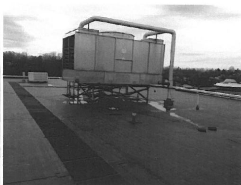
After Photo - New Roof with Walking Pads
