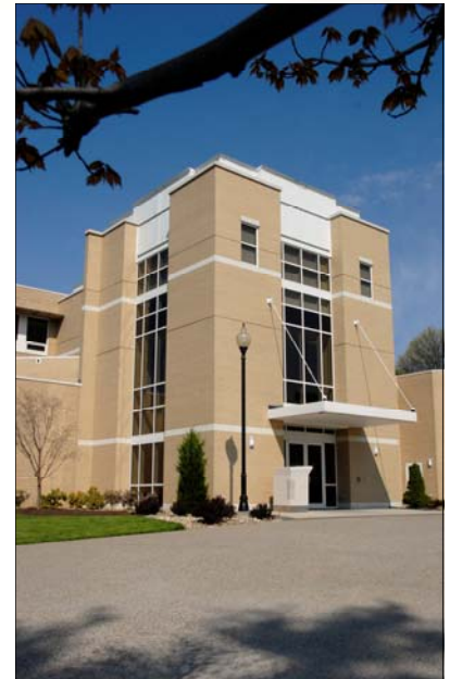
Ruth Ann Musik Library Renovations & Additions at Fairmont State University Fairmont, West Virginia
