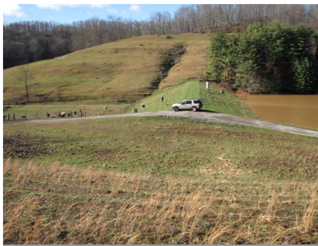
Salem Fork Site 11A. Gannett Fleming evaluated several spillway rehabilitation alternatives to comply with Class C high hazard design criteria and recommended armoring the auxiliary spillway.
