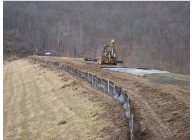
Figure 26: New Creek Site 14 Pollution Control Measures. We inspected erosion control measures for the access road along the crest of dam for the multi-year construction project at New Creek Site 14.
