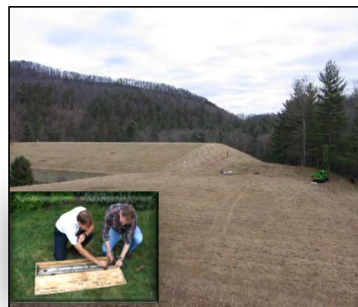
Figure 5: Lake Laura Dam. Our geologists and geotechnical engineers performed subsurface exploration and mapped the geologic profile of the auxiliary spillway at Lake Laura Dam to develop the erodibility parameters needed to evaluate the stability and integrity of the auxiliary spillways.
