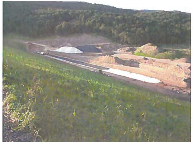
Figure 27: New Creek Site 14 Fine and Coarse Drain Fill Placement. Our experienced fill/excavation inspectors were on site during placement of fill/drainfill at New Creek Site 14.
