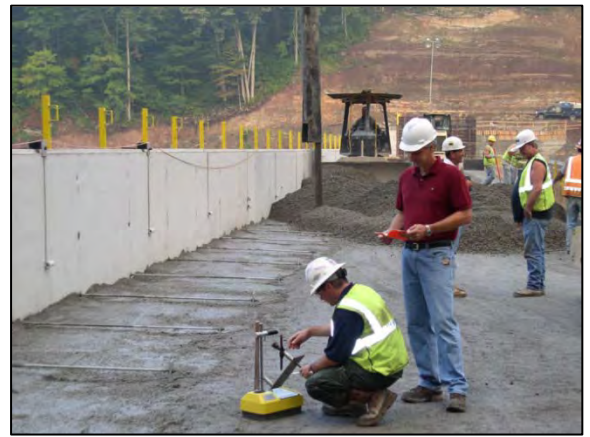
Figure 23: Elkwater Fork Dam. Gannett Fleming oversaw quality control testing of RCC at NRCS WV's Elkwater Fork Dam.
