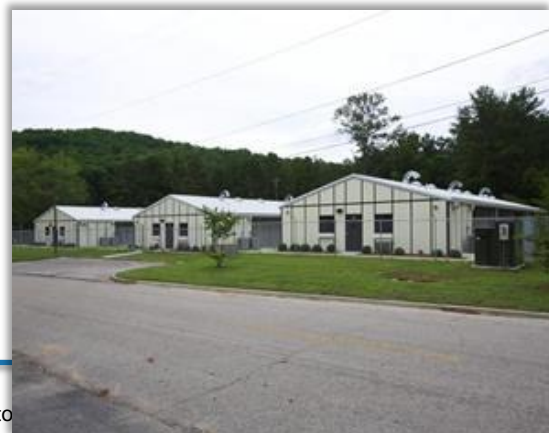
Figure 1-2: Training Facility Kennels
