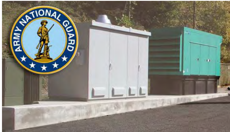
Emergency Generator Stations
