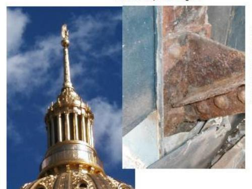
The structural steel in the lantern level shows evidence of deterioration. Project included probing to determine extent of deterioration and preparation of plans and specifications for repairs.
