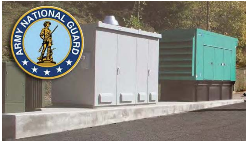
Emergency Generator Stations
