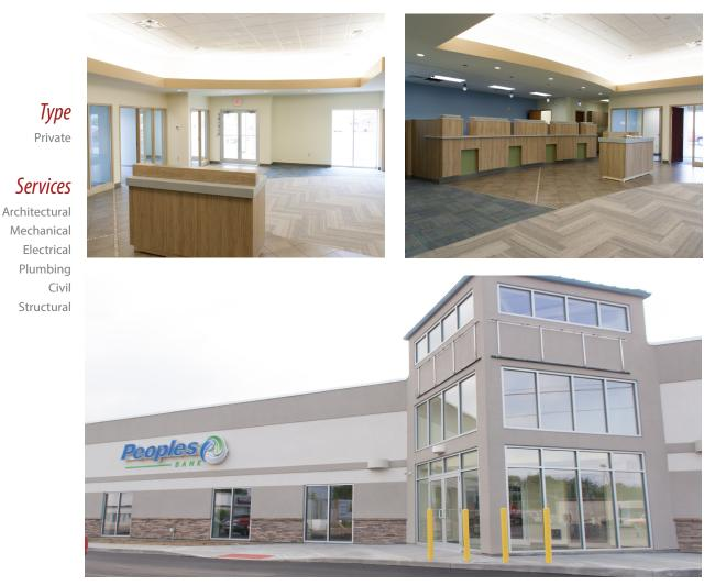
This project was to renovate an existing 12,000 SF office building into a 6,000 SF retail banking branch. Half of the existing building was demolished to make room for the new drive through lanes. A new entry tower was constructed, and exterior finishes were updated throughout. Work was performed through multiple prime contracts.
