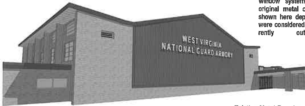
Existing Metal Facade
