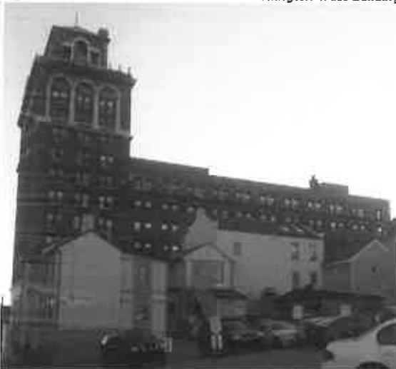
McKinley & Associates' Washington, PA Office
