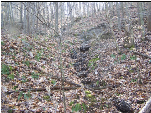
Eroded drainage path from bench
