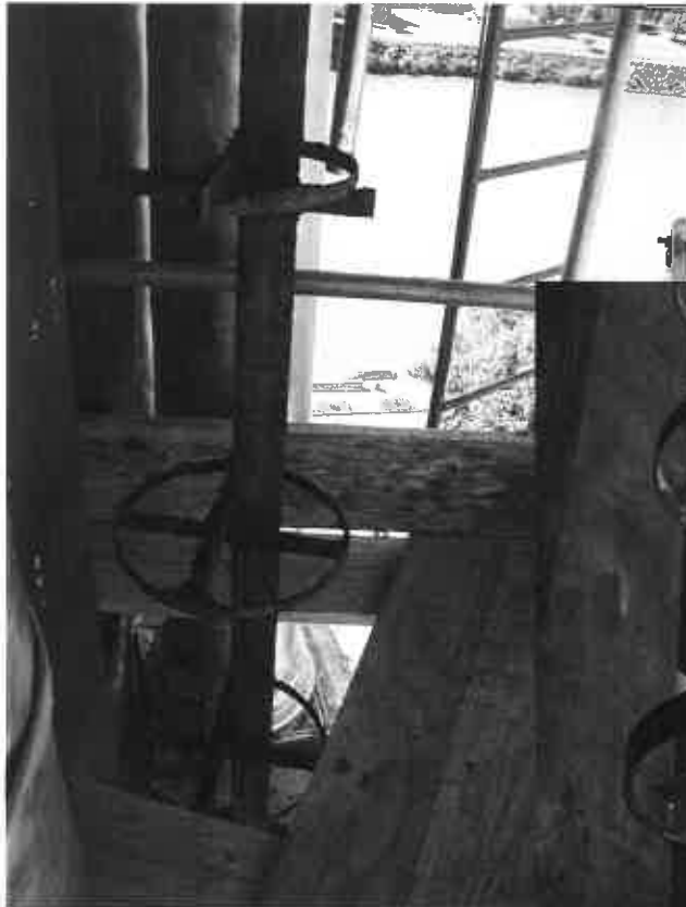
Removal of one decorative column wrap indicated that back-up structure was severely deteriorated. Members were replaced with new galvanized components.
