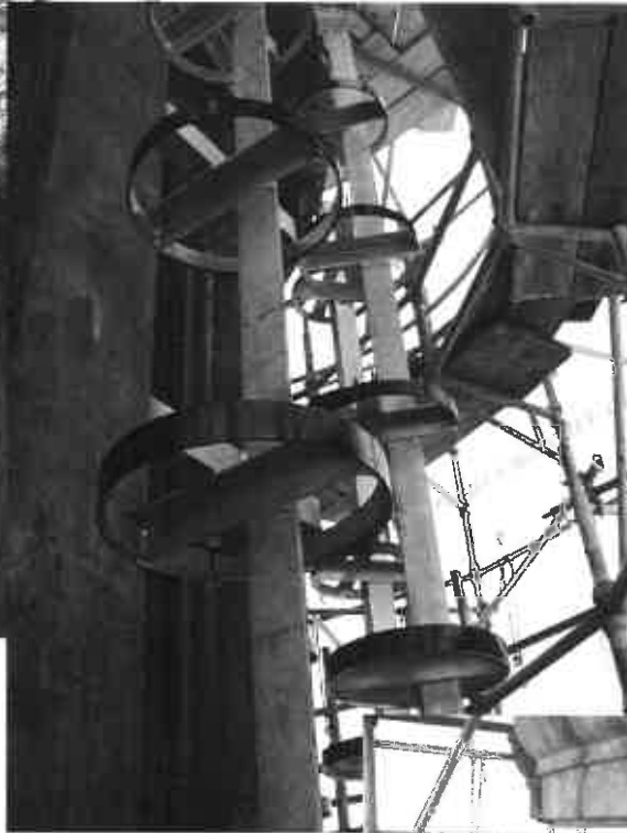
Removal of one decorative column wrap indicated that back-up structure was severely deteriorated. Members were replaced with new galvanized components.
