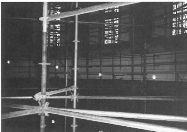
Photo during construction
