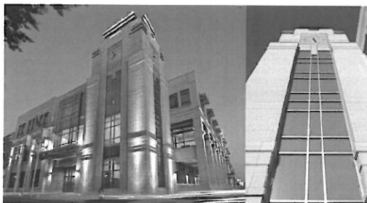
Raleigh County Judicial Center AIAAW Merit Award for Achievement in Architecture 2013
