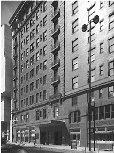
PWWG's comprehensive restoration of the National Register 21c Museum Hotel in Cincinnati included removal of 1 elevator, upgrades to 2 others, and replacement of an existing manually operated elevator with a new service elevator.
