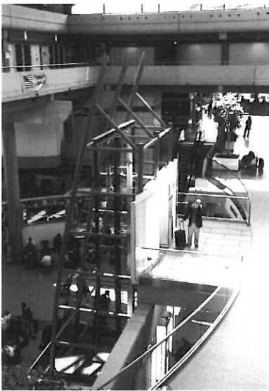
PWWG's retrofit Landside Elevator at Pittsburgh Int. Airport is a partial steel and glass enclosure with no shaft. The steel pipes of its fully exposed frame are sympathetic to the steel trusses that form the vaulted roof structure of the space.
