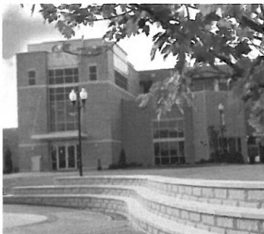
Tower Engineering completed a comprehensive elevator modernization and systems upgrade at the Ruth Ann Musick Library at Fairmont State.
