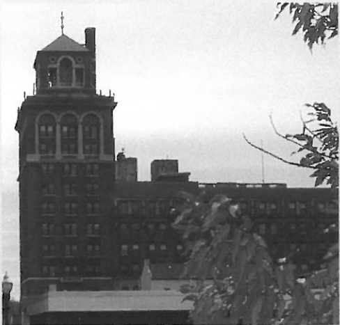
McKinley & Associates' Washington, PA Office
