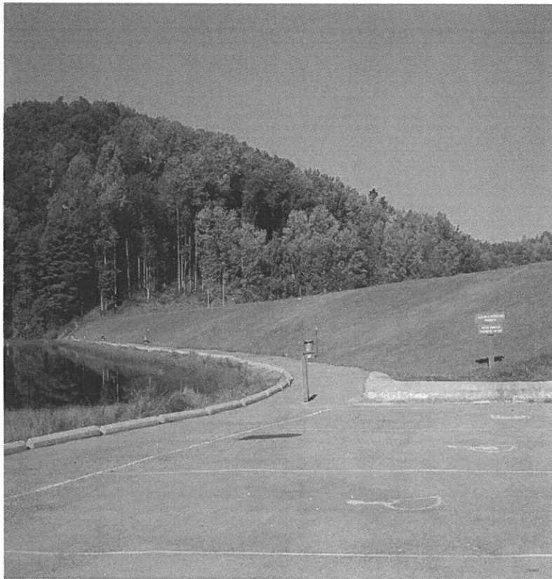
TETER CREEK DAM MODIFICATION, BARBOUR CO., WV
