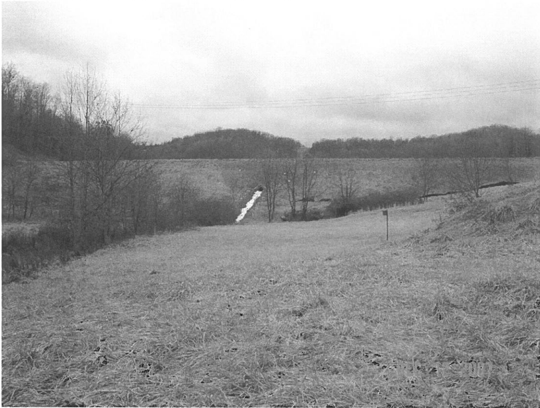
LEMLEY DAM MODIFICATION, MONONGALIA CO., WV
