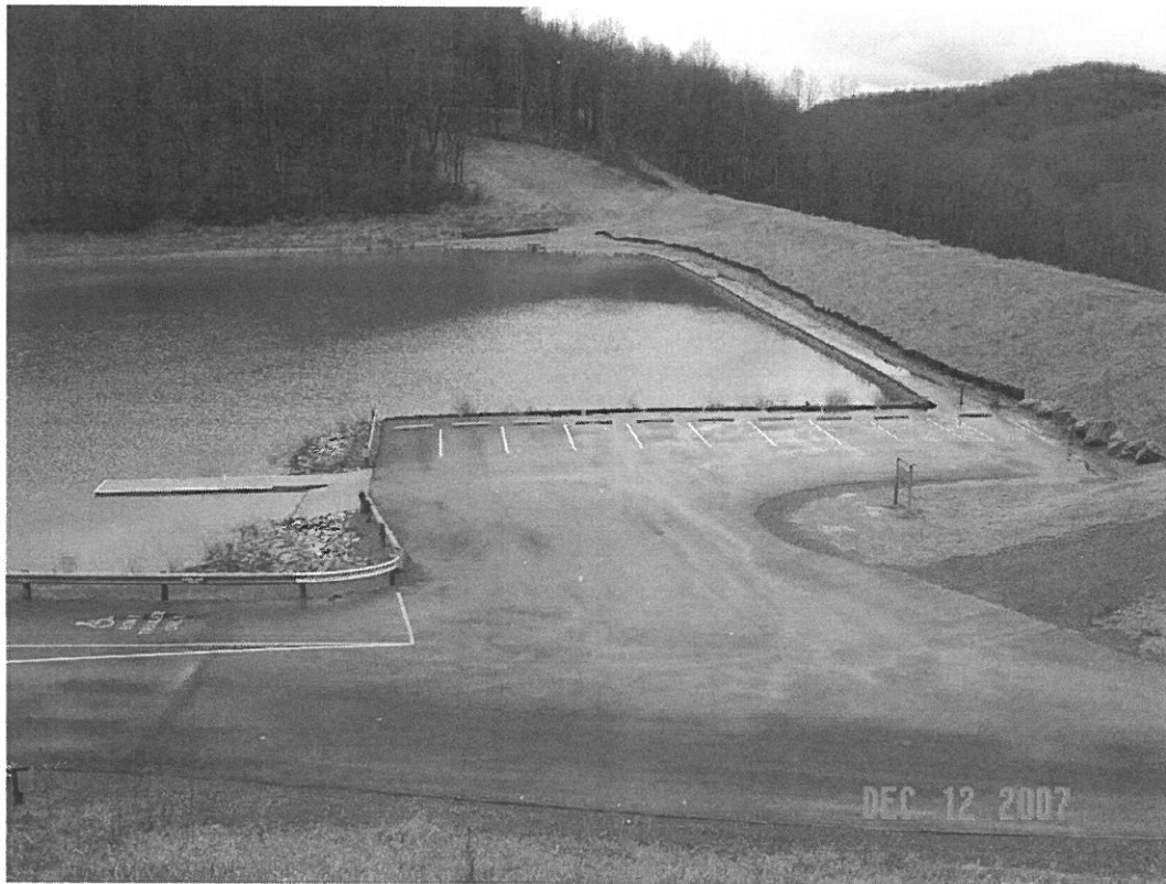
BAILEY DAM MODIFICATION, MONONGALIA CO., WV
