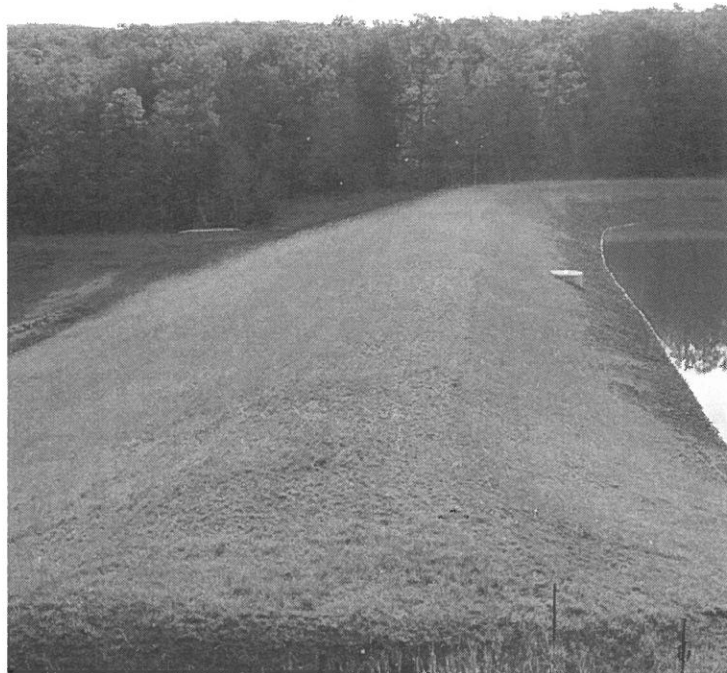
WILSON DAM MODIFICATION, HAMPSHIRE CO., WV
