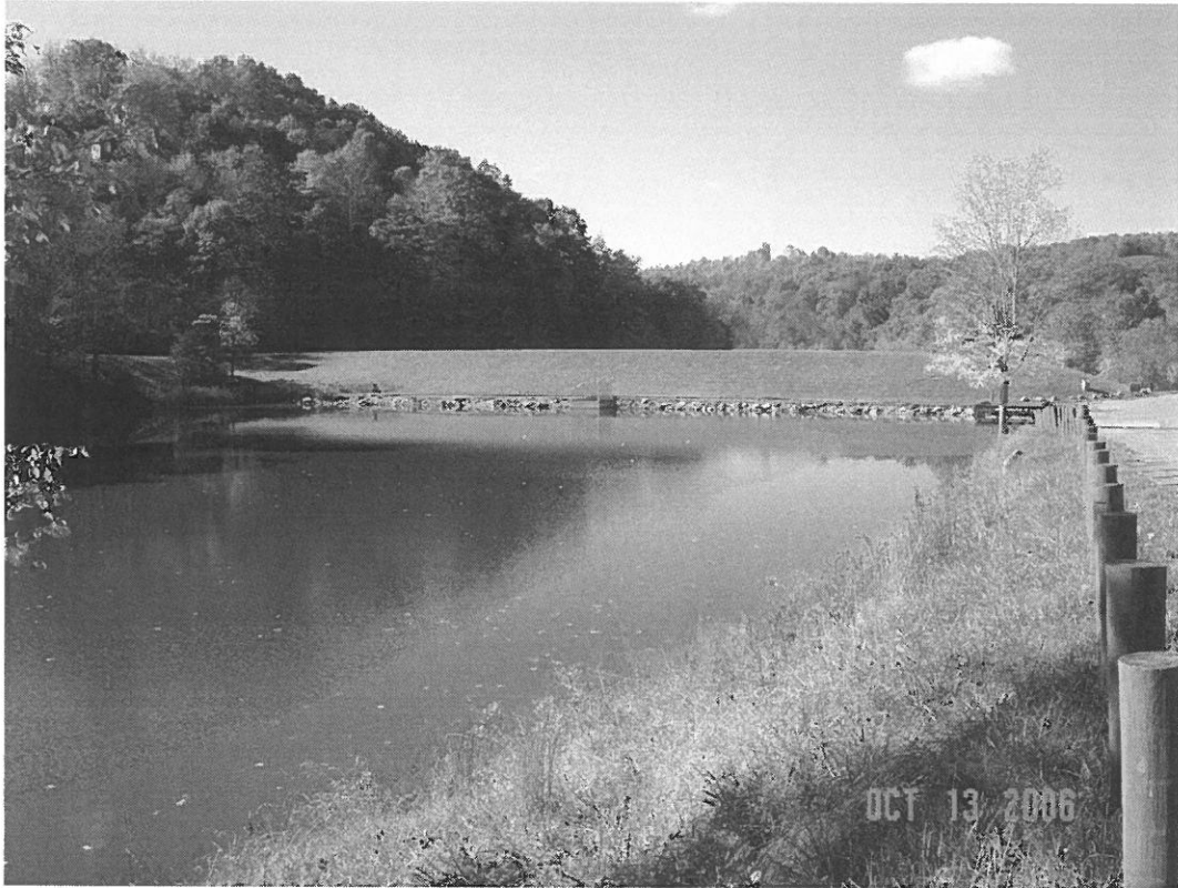
JIMMY LEWIS DAM MODIFICATION, MERCER CO., WV
