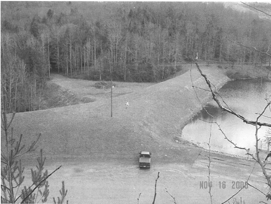
PLUM ORCHARD DAM MODIFICATION, FAYETTE CO., WV
