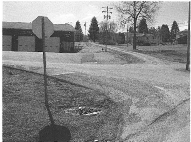
New Storm Drains and Catch Basins
