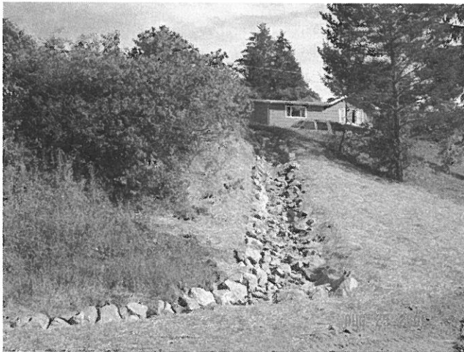
Erosion Repair – Rip Rap Armored Ditch
